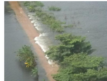
FIGURE 2.11 FLOOD OVER A ROAD/CEM ROAD
