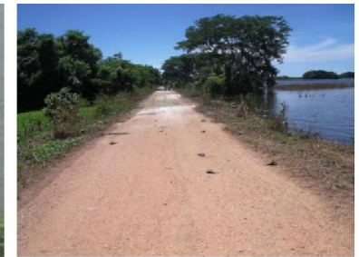
FIGURE 2.12 NO DAMAGE AFTER A FLOOD ON THE ROAD
