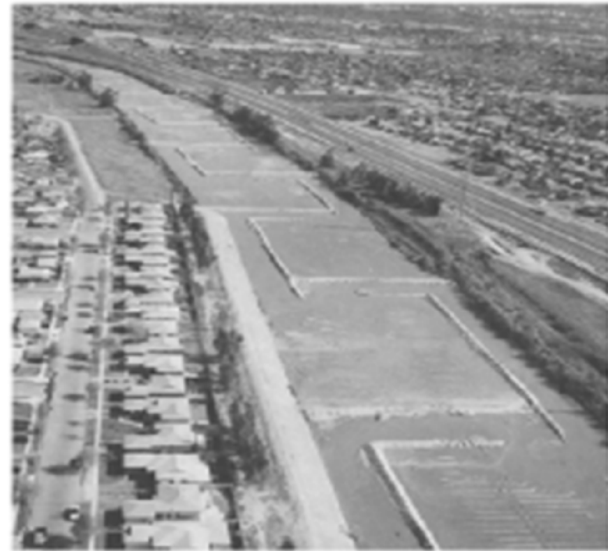
Finger Levees in San Gabriel River below Whittier Narrows Dam, California. Photo courtesy of Los Angeles County Flood Control District.
