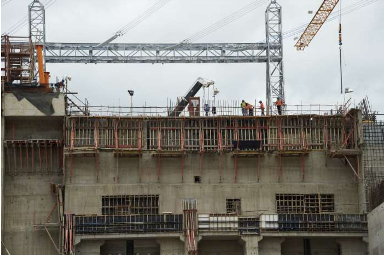
Workers are standing on a dam in Lao PDR that is under construction.
