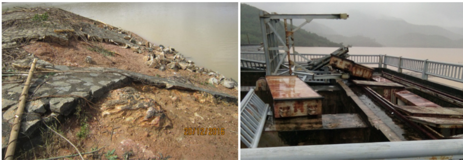
Fig. 6. Damages to the Van Hoi dam and its facilities due to landslide-generated waves (Photo courtesy by Do Canh Hao).
