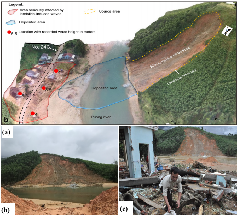
Fig. 4. (a) 3D view of the Tra Giang landslide [59]; (b) Landslide after sliding (photo by Dinh Thi Quynh); and (c) Collapsed houses due to tsunami waves [63].
