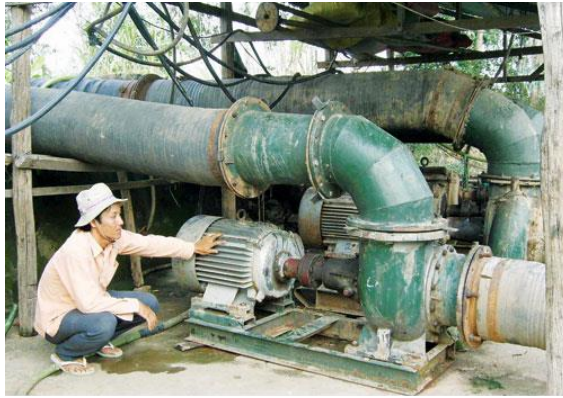
Pumping station in the M.D
