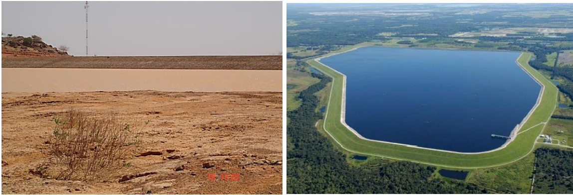
Off-river reservoirs in Burkina Faso and in USA
