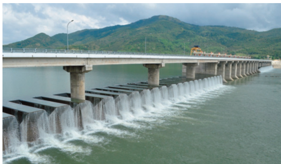
Figure 3. Van Phong dam spillway with a 5 m high type-A Piano Key weir in Vietnam (commissioned in April 2015). Photo courtesy of VNCOLD.
