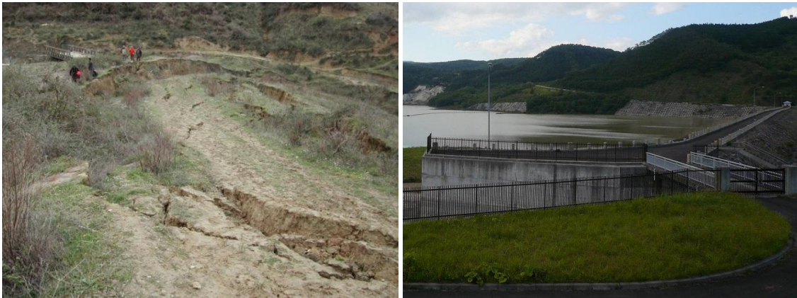
Figure 4. Failure of Sharredushk embankment dam in Albania due to a magnitude 4.1 earthquake in 2009 (left) and undamaged Aratazowa rockfill dam in Japan, which was subjected to peak ground acceleration of 1.0 g during the magnitude 7.2 Iwate Miyagi Earthquake in 2008 (right)
