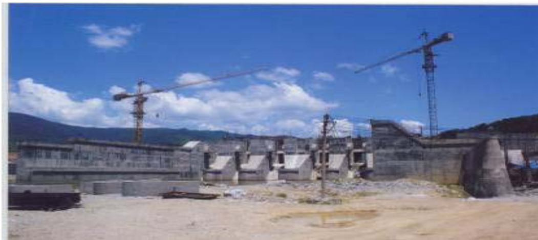
Downstream Slope of the Dinh Binh RCC Dam
