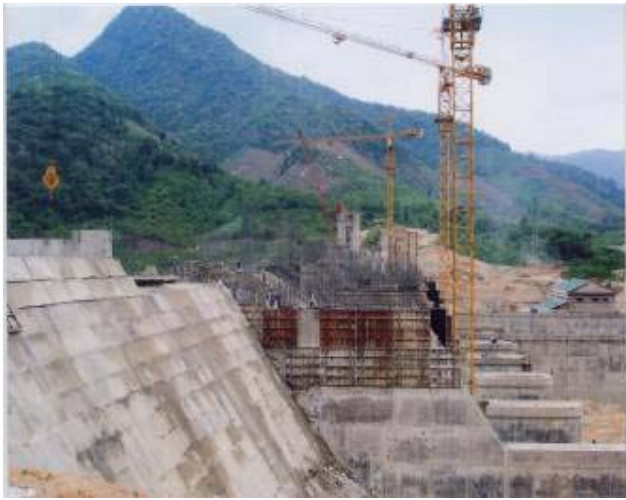
Downstream Slope of the Dinh Binh RCC Dam
