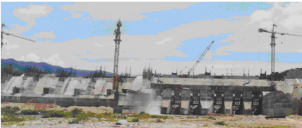
The RCC dam is under construction
