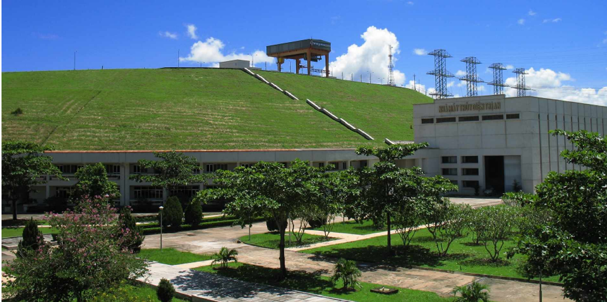
Tri An Hydropower Plant in the South Vietnam, 400 MW power capacity, 2.7 km 3 water storage reservoir
