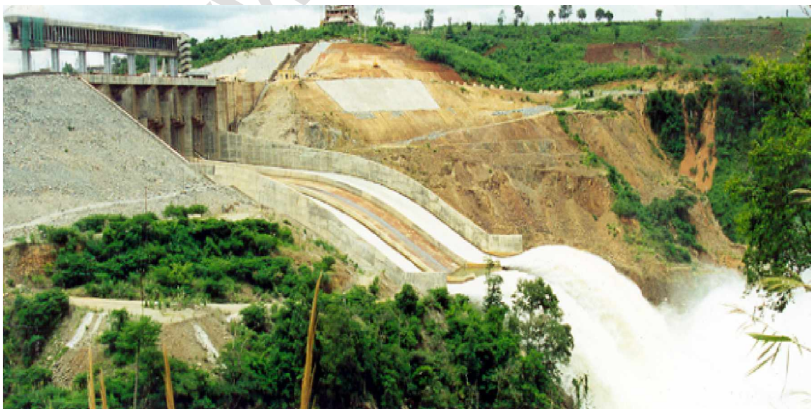
Yaly Hydropower Plant in the Western Highland of Central Vietnam, 720 MW
