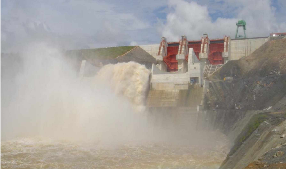
Dai_Ninh Hydropower Plant in the Southern part of Central Vietnam, 300 MW
