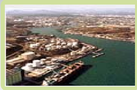
National Industrial Complexes
