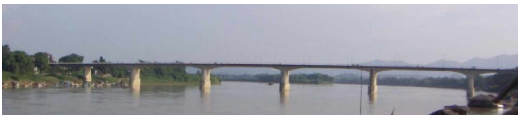
The Lo River Bridge in Tuyen Quang Town
