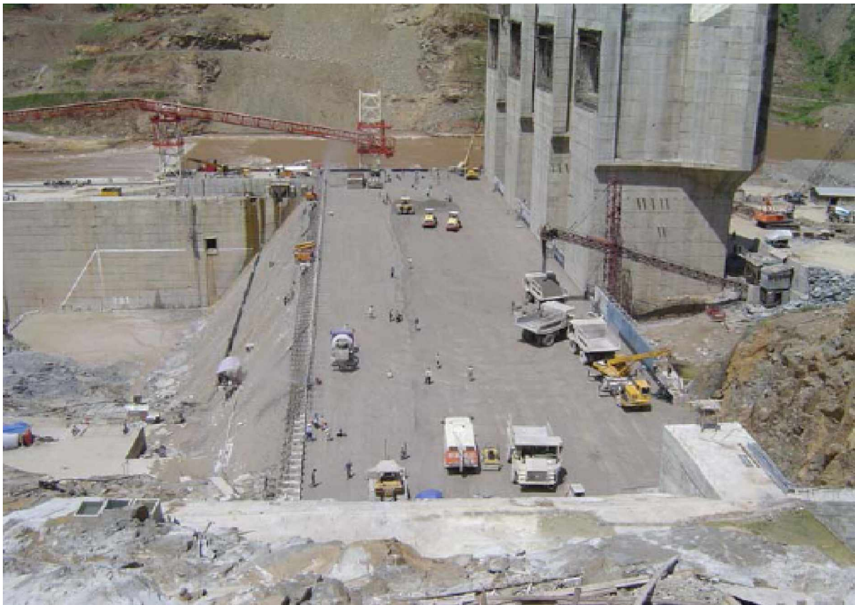
RCC Placing Stage 4a
