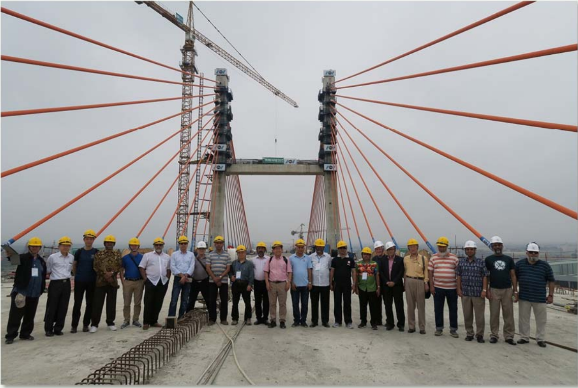
Photo 3: Group photo on Bach Dang Bridge (under construction)
