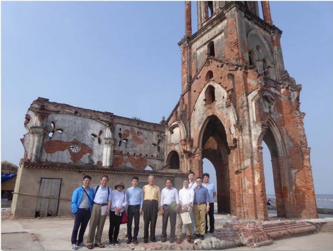
Photo 5: A Church Ruined by Coastal Erosion and Typhoon, Hay li, Nam Dinh Province, Vietnam
