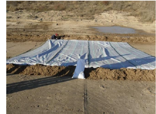
3. Covering with Vegetation Mat
