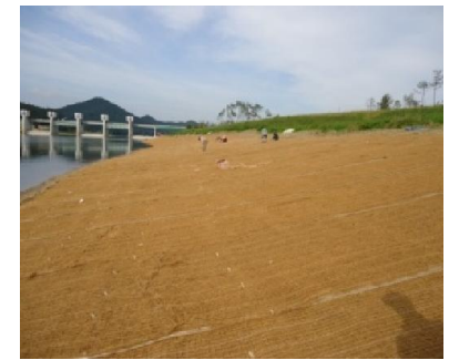
<Installation of Vegetation Mat>
