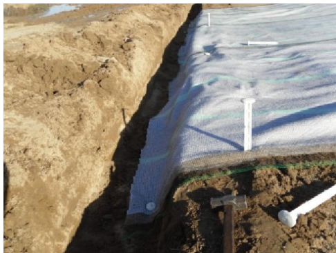
4. Fixing Pin Installation
