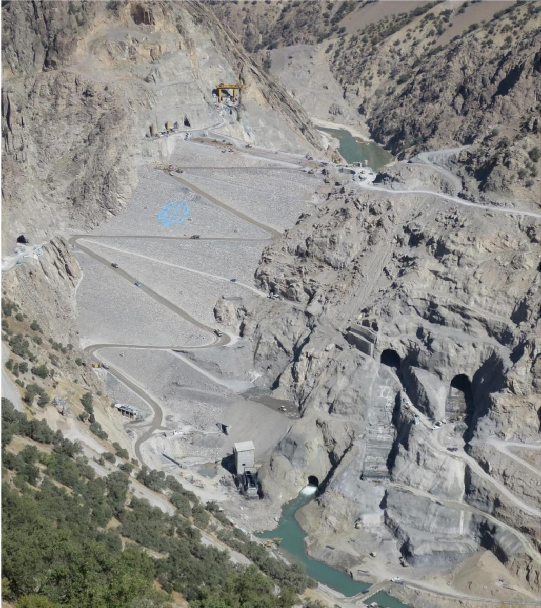
Figure 2. Downstream view of the ongoing construction works of the Rudbar Lorestan earth core rockfill dam, which is located in an area of high rockfall hazard and strong earthquakes. On the left bank the two spillway tunnel portals and the outlet of the diversion tunnel are visible.
