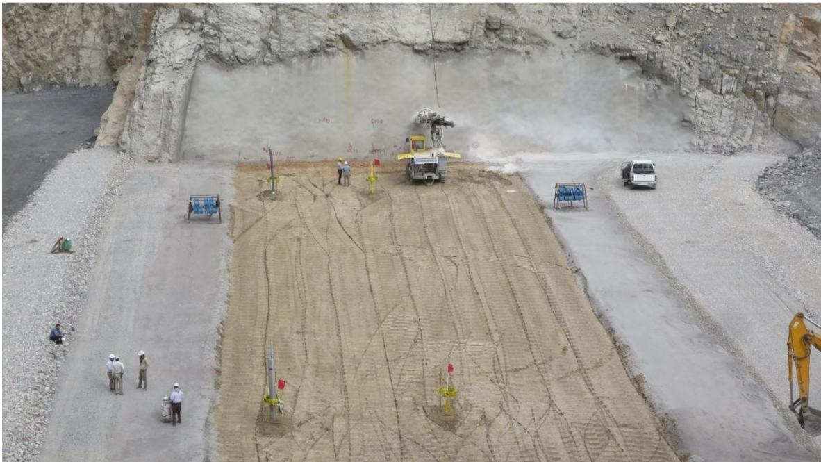
Figure 1. View of core, filter and transition zones in ECRD located in a narrow canyon with multiple discontinuities in the footprint of the dam. The fine sand filter is flared towards the abutment
