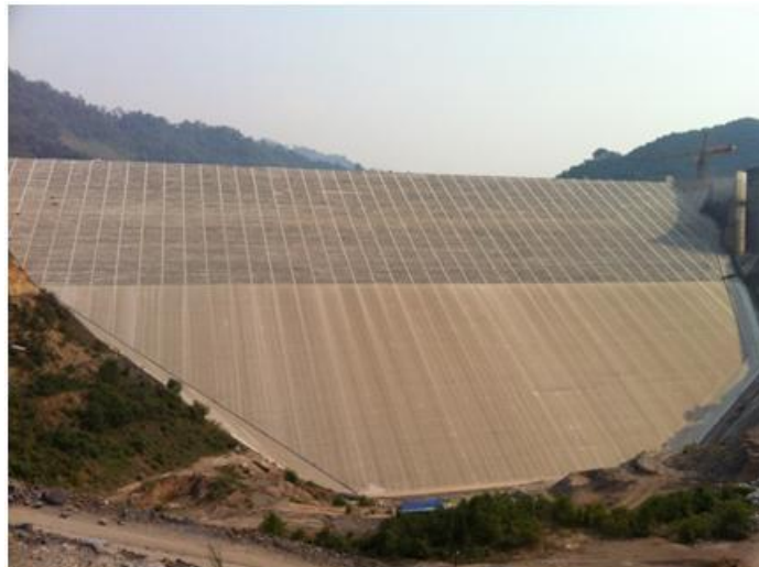
Figure 1: Nam Ou 6 dam, 88 m high, with upstream PVC facing commissioned in 2015
