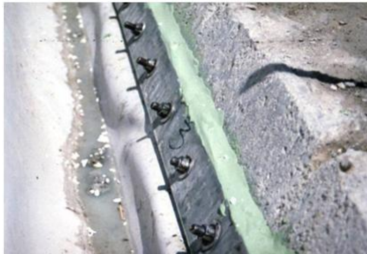
Figure 16: The mechanical watertight fixation of the composite to the concrete plinth
