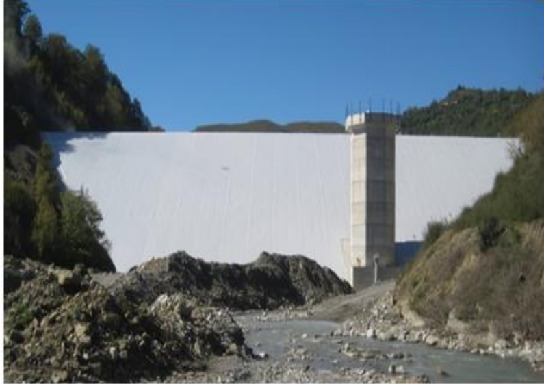
Figure 3: Murdari GFRD dam waterproofed with wide, pre-welded, bands of polymer 'composite': PVC geomembrane + PP geotextile.
