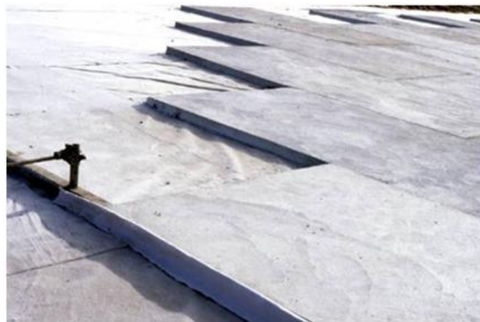
Figure 21: Medium unreinforced, cast in place concrete slabs protection
