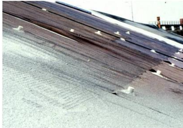
Figure 20: Light geotextile + shotcrete protection on a relatively flat slope
