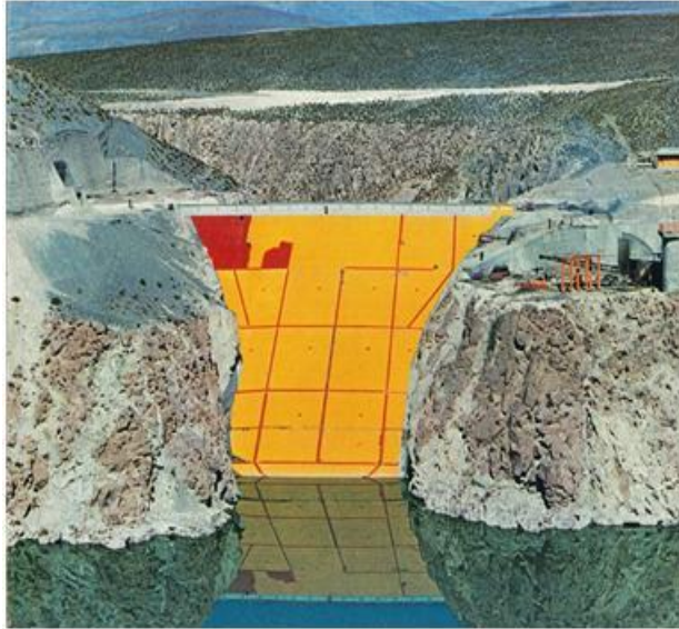
Figure 2: Aguada Blanca ingot iron faced rockfill at 3640 m altitude in the Andes
