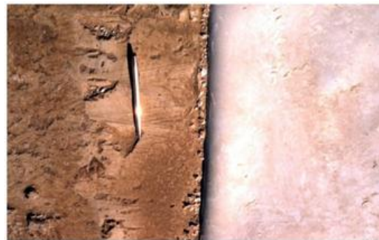
Figure 18: Close-up of a training ‘insert’ fixation (left) and an ‘insert’ on the top of a plastic concrete cut-off (Jibiya dam) (right)
