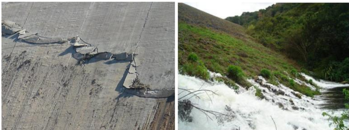
Figure 4: Damage to a concrete facing due to rockfill deformations (left) and large water loss crossing the embankment, consequence of invisible damages to the facing (right).
