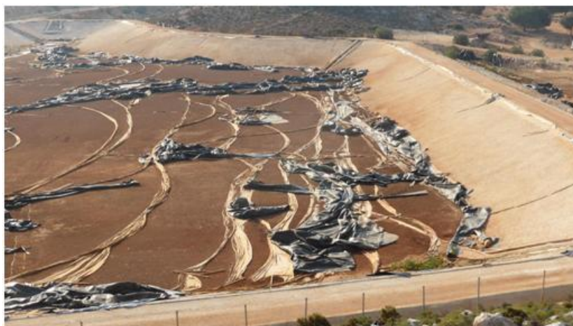
Figure 23: Total destruction of the geomembrane and of the underlying geotextile by wind. Anchors were not installed
