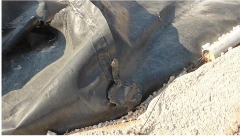
Figure 13: Elongations and distresses of an HDPE liner produced by temperature changes
