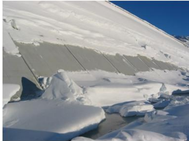
Figure 11: A PVC 'composite' facing under severe winter conditions (Norway)
