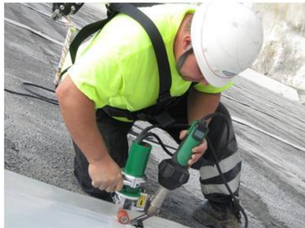
Figure 14: (left) Modern automatic, double track and (right) single track, hand-held welders (courtesy CARPITECH)
