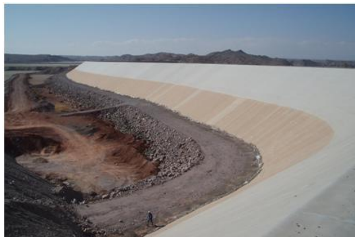
Figure 10: A staged application of a geomembrane facing on a tailing dam in hot climate (Iran)
