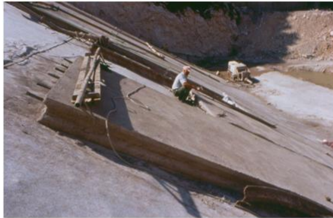
Figure 22: Heavy cast-in-place concrete slab protection. Reinforcing steel may be necessary on some slabs and dowels may be required along some joint
