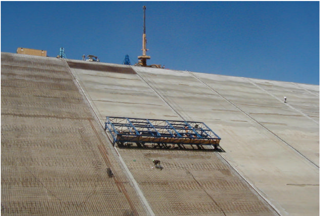
Photo 3. Reinforcement placing trolley
