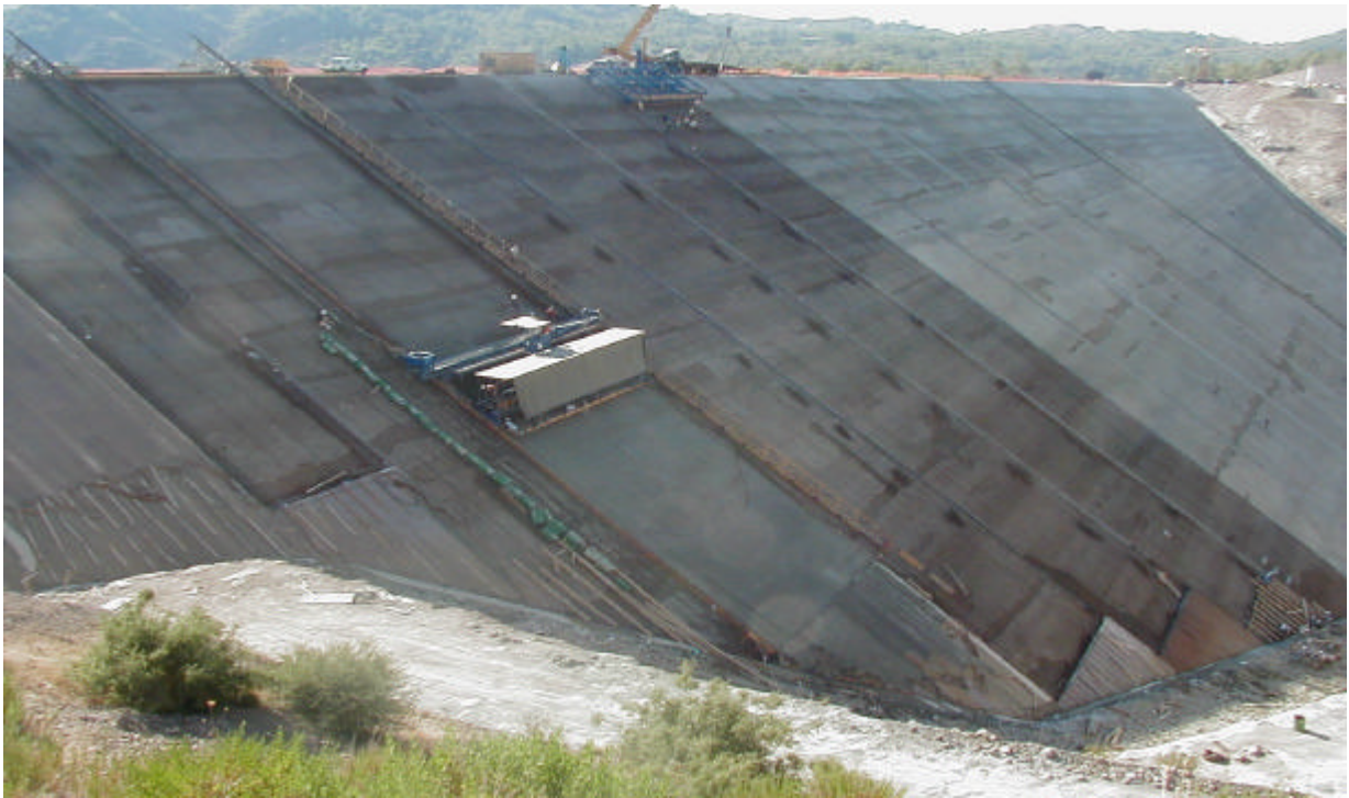
Photo.1 Upstream Face Slab Concreting
