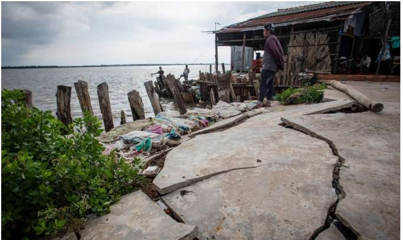
What's left after a house collapses into the river due to erosion in Soc Trang Province, partly caused by dam construction on the Mekong River, July 2019.
