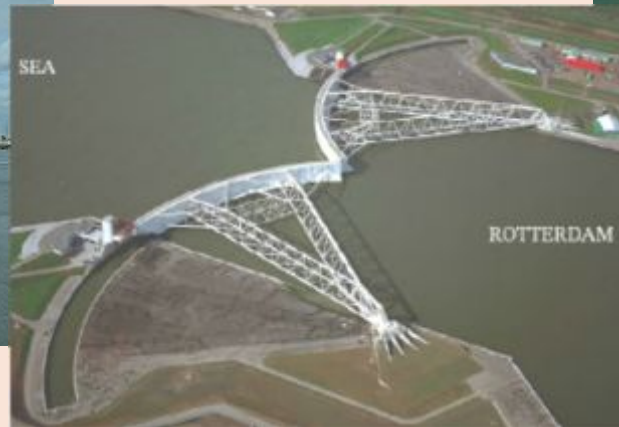
Maeslant Storm Barrier (NL)
